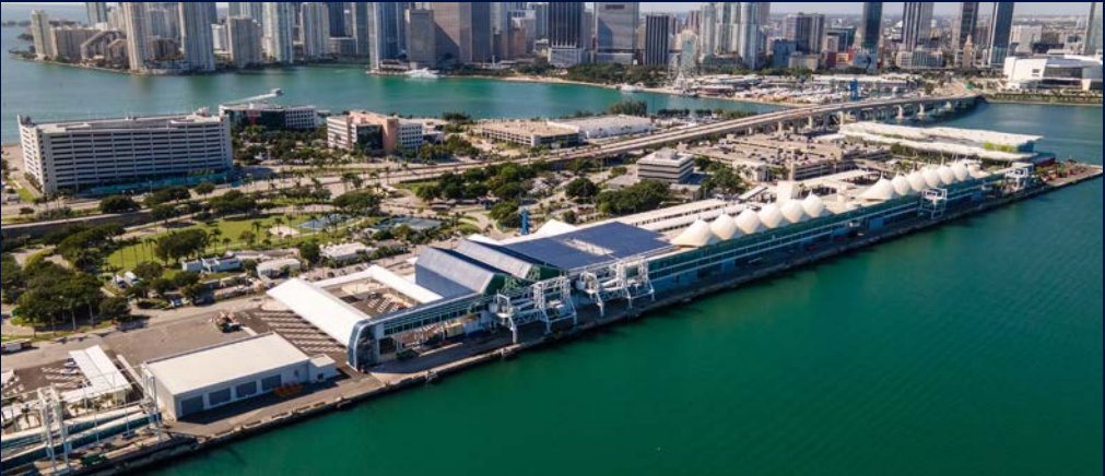
PortMiami Terminal F Renovations - Miami, FL
