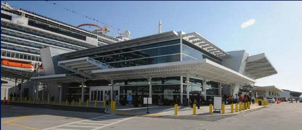
PortMiami Terminal D Expansion - Miami, FL
