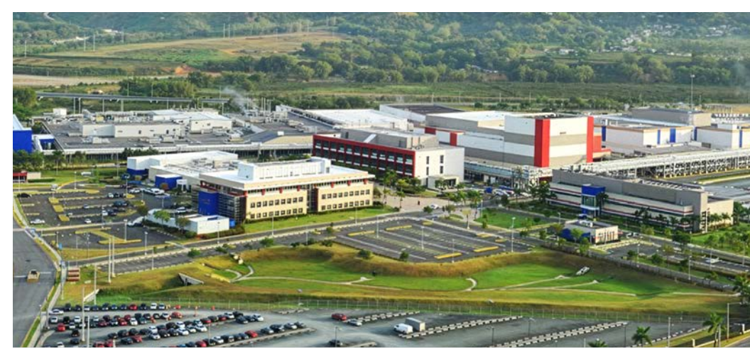
Amgen Manufacturing Limited, Buildings AML 6 and 14*
