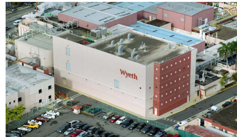
Wyeth Pharmaceuticals Parenteral Building D Expansion*
