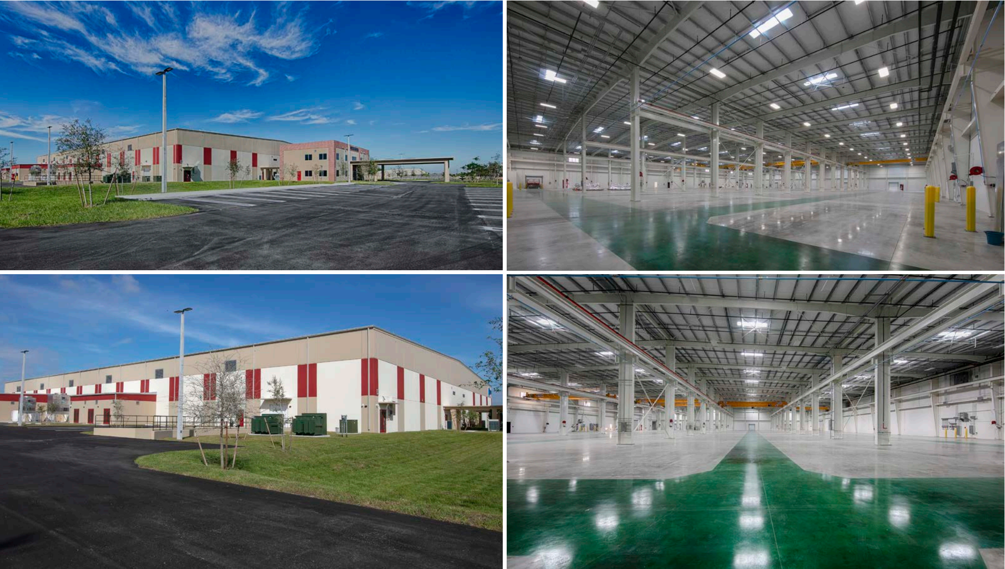
This image features ZERO ARTIFICIAL lighting. Structural standing seam roof with the prismatic skylights (PRISMAX) result in very low energy consumption.
