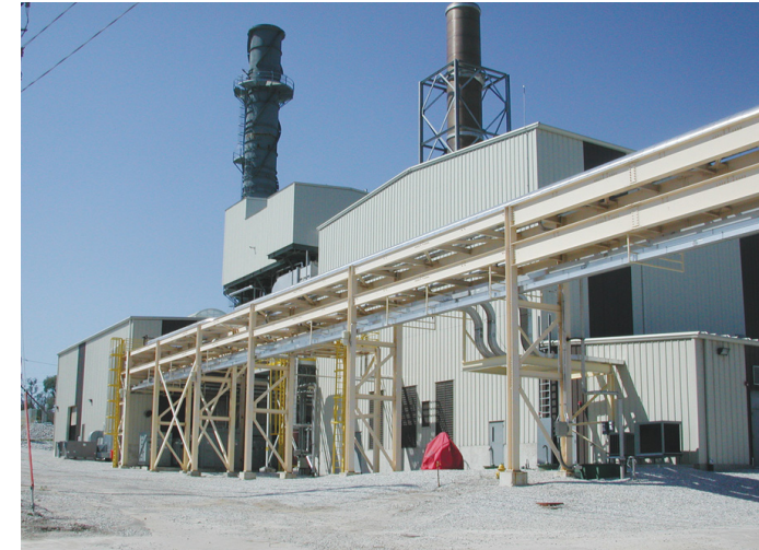
Roquette America, Inc., Co-Generation Facility - Keokuk, IA (Courtesy of VP Buildings)
