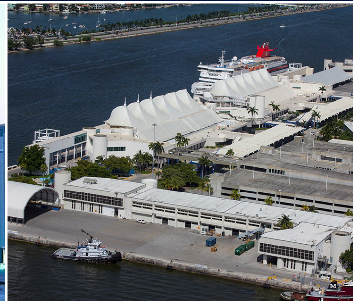
PortMiami Command & Control Center (C3) – Miami, FL
