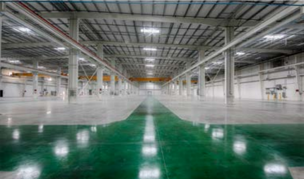
This image features ZERO ARTIFICIAL lighting. Structural standing seam roof with the prismatic skylights (PRISMAX) result in very low energy consumption.
